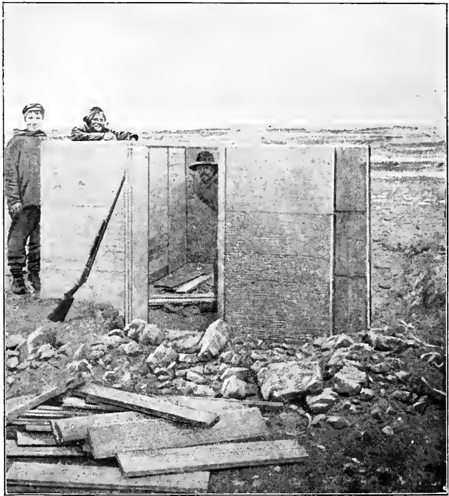
BUILDING THE MAGNETIC VARIATION HOUSE. GJÖAHAVN, 1903.
